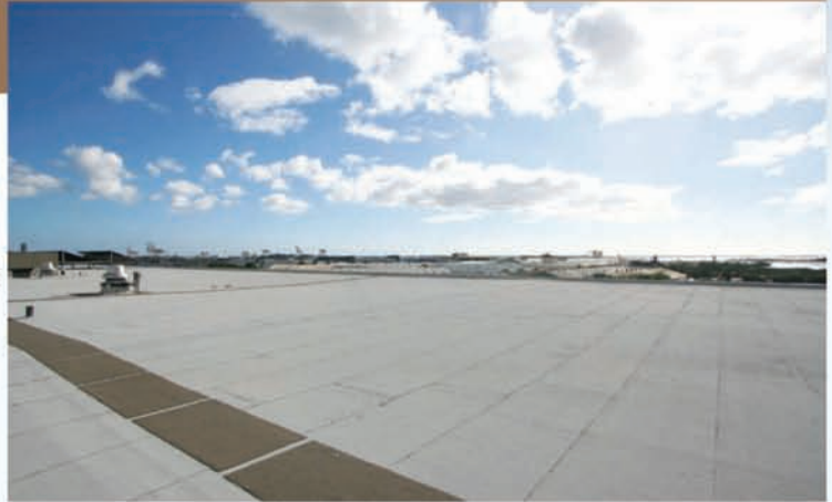
Completed in late 2011 was the complete tear-off and reroof of the First Hawaiian Bank building in the Kamehameha Industrial Center.
